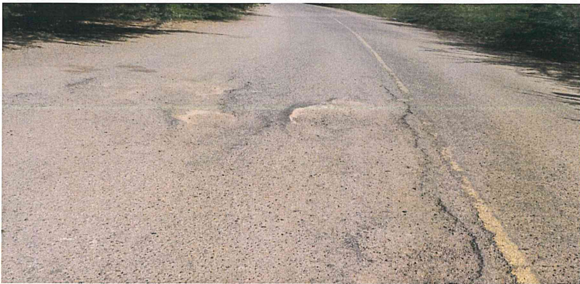
Photo 10: Malka Suftu Road: fretting and potholes at km 1+420
